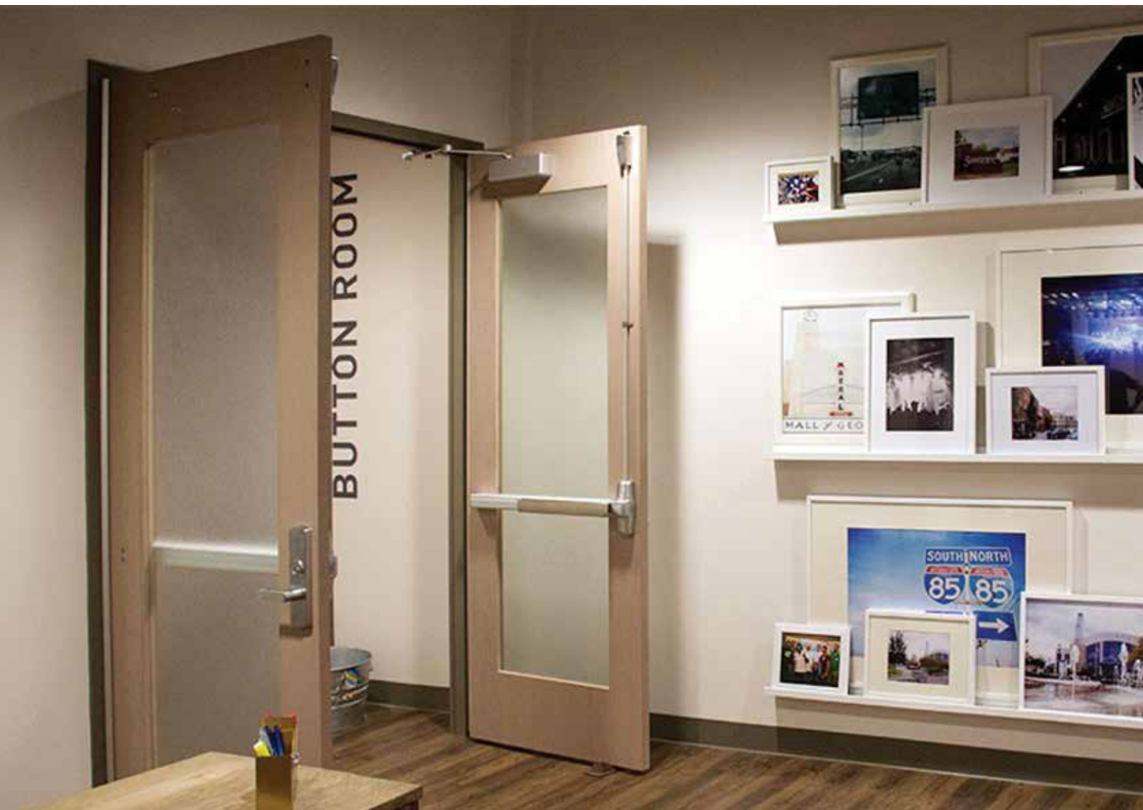
A pair of doors with full light cutout and exit device is finished in a custom stain color.
